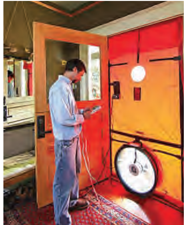
Technician performs a blower door test to analyze how leaky this house is and where air sealing would be most effective.
